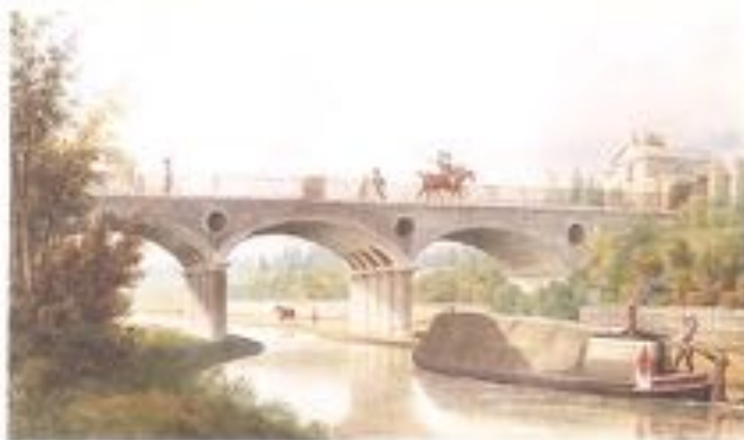
Maidenhead Bridge, Robert Rail Barred after Company's chairman, the Earl of Maidenhead. Shows the canal in cutting on the north side of Roper's Park. 1 m. (right), 1835. courtesy of Alan Foxwell
